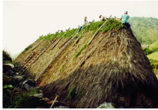
Thatching a roof.
